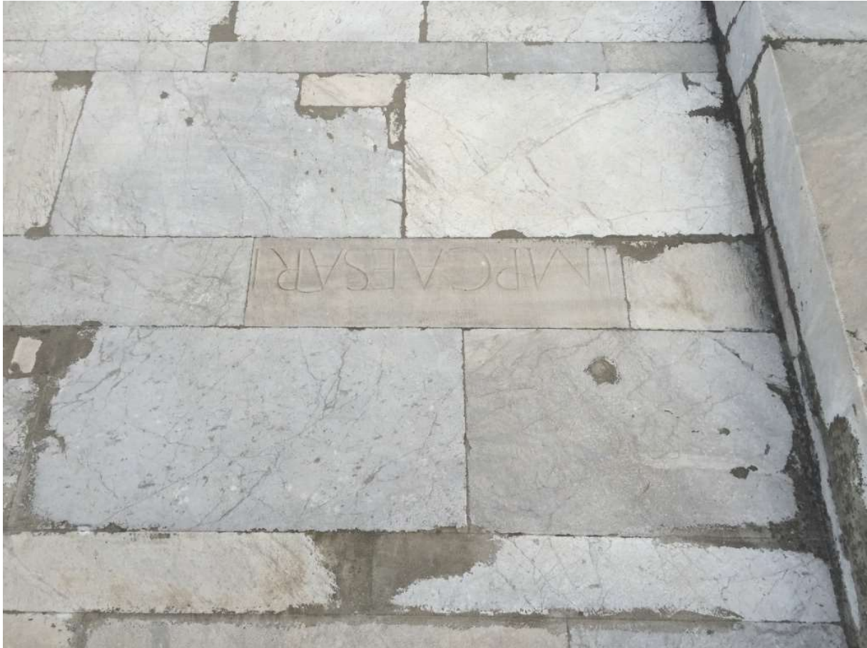
Illustration 1 : Reuse of Roman building materials as exemplified by the Cathedral of Pisa (Photo ©Marcos Buser).
